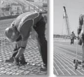
Instead of tying Rebar by hand try using a Rebar-tying tool with an extension handle
